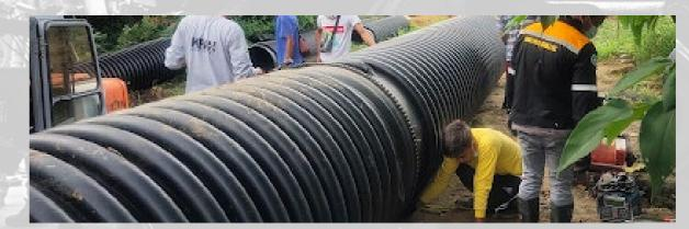
The wire is heated with the help of a fusion device whereby the two pipe ends
