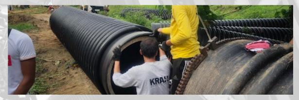
Additional advantages include the ability to install in small trenches without the use of heavy equipment and quick piping installation due to the simultaneous use of numerous fusion devices. The final joint is a tight one that is permanently attached.
